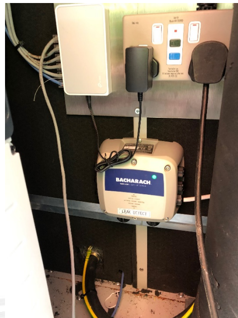
The leak detector fitted to the CO 2 compressor pack
