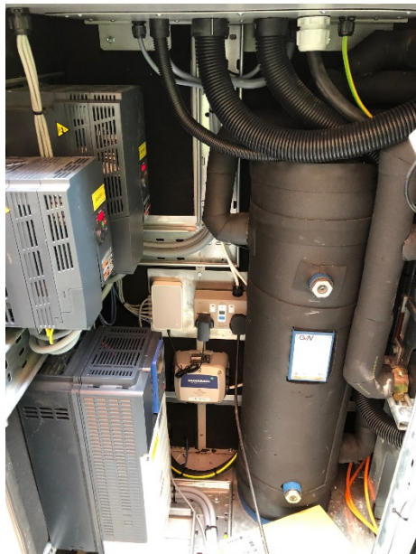
The leak detector fitted to the CO 2 compressor pack
