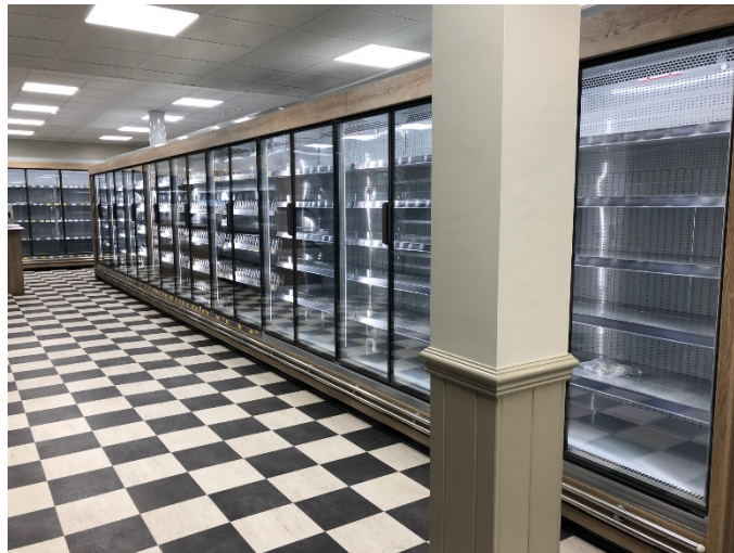
New cabinets installed at Lincoln Co-op
